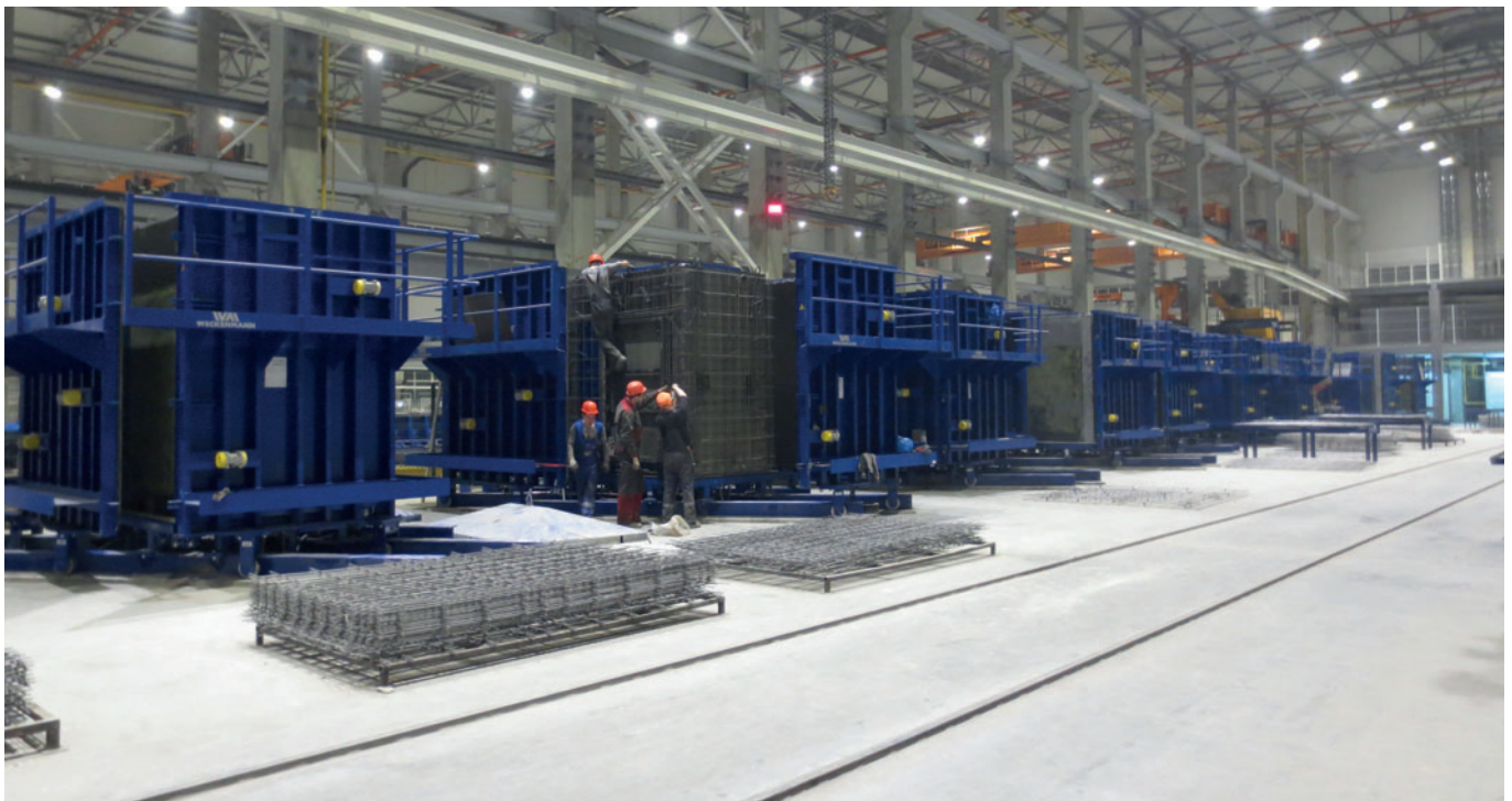
Inline lift shaft formwork
