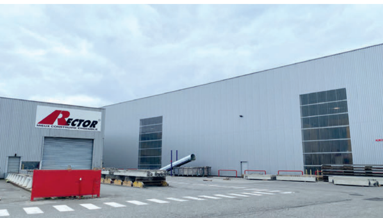
hall with second circulation system for manufacturing double and element floors
