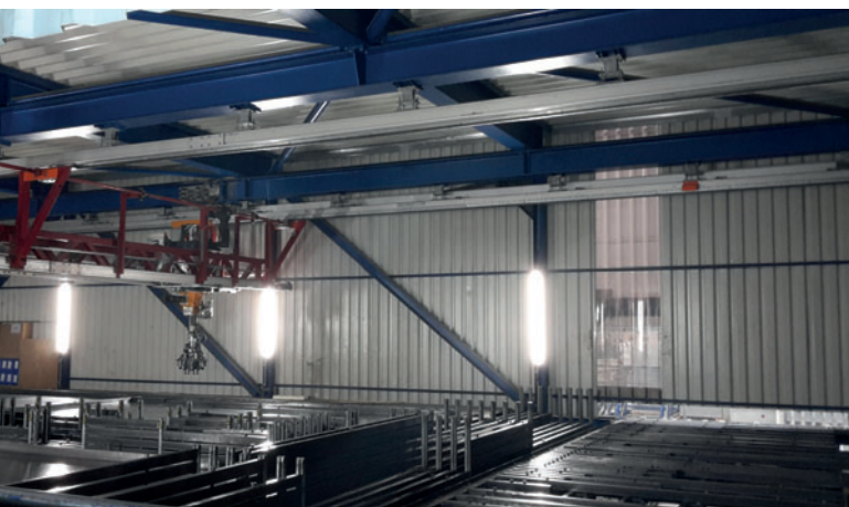
Before retrofit project: Formwork plant at ABI Bedburg
